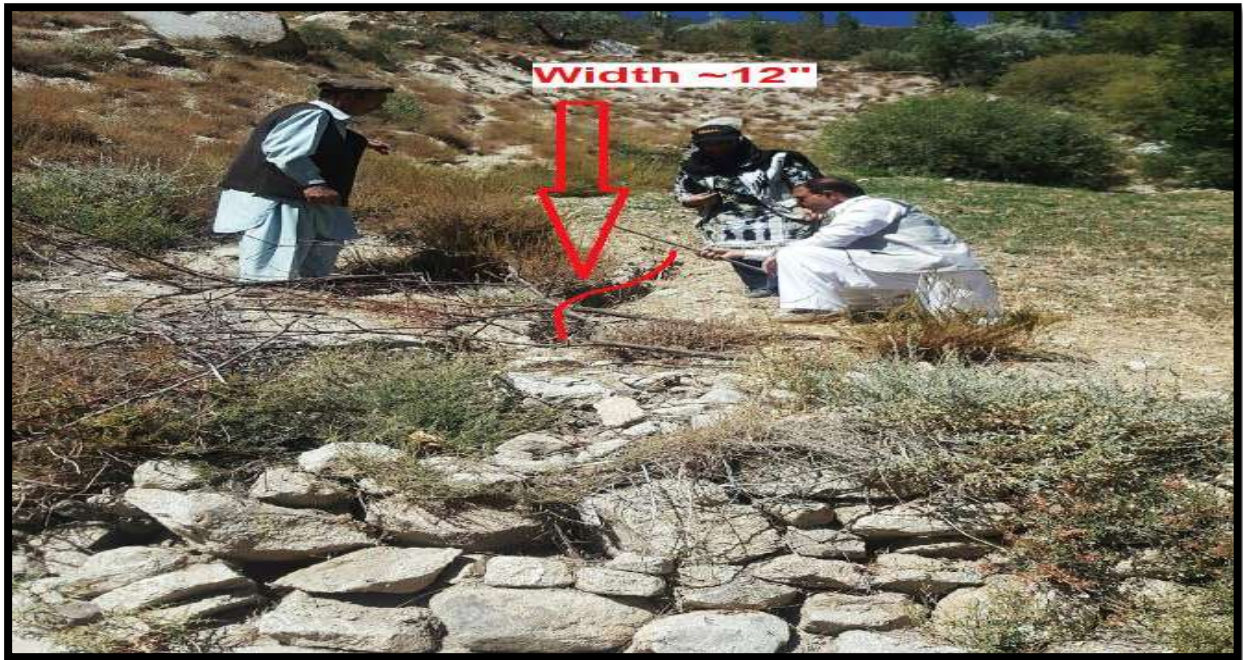
Figure 8: Team Observing width of Crack in the Valley
