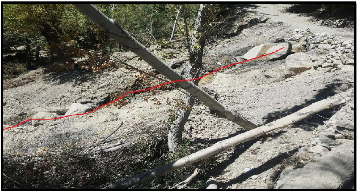
Figure 7: Visible Cracks observed during Field Visit
