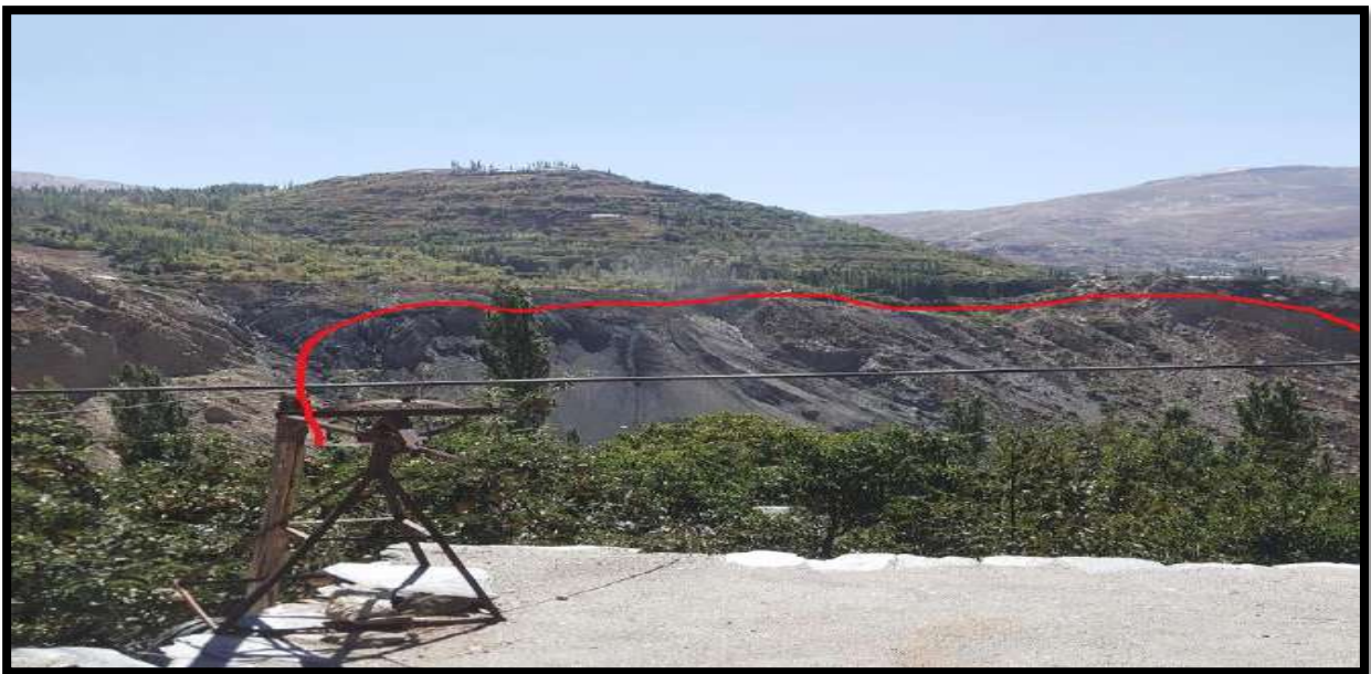
Figure 9: Debris Flow observed during Field Visit
