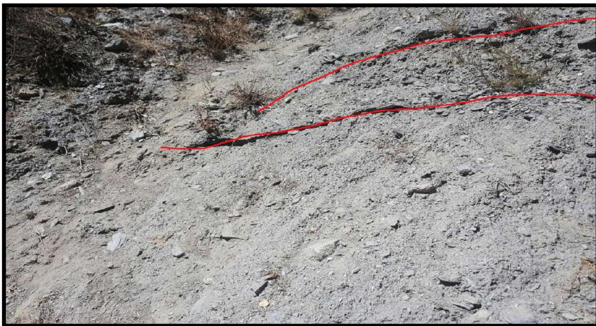
Figure 11: Cracks observed at different locations in the Valley
