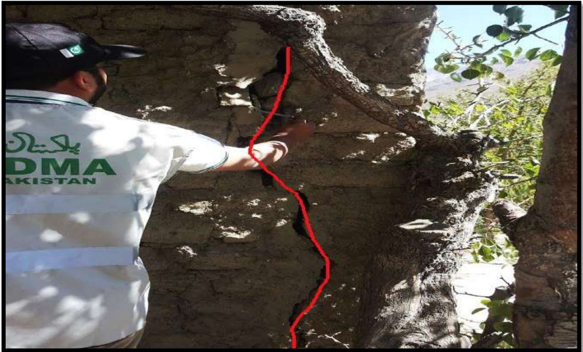
Figure 14: Damaged Cattle Sheds due to continuous landslide events
